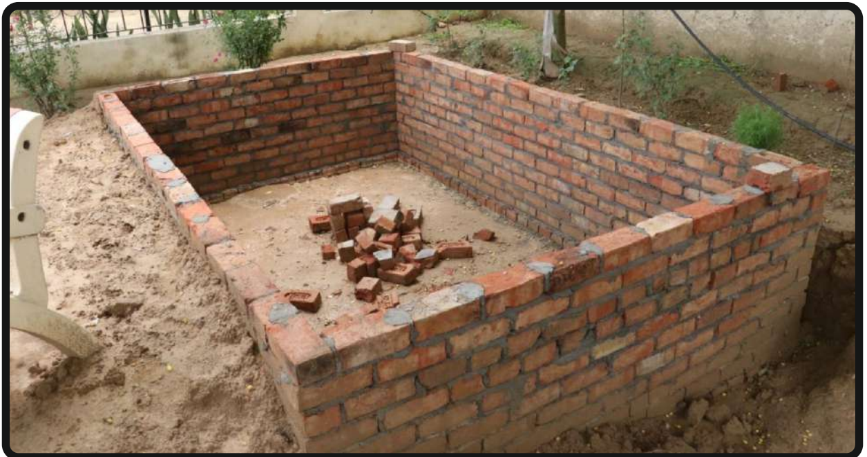
Pit for compost making and organic waste disposal
