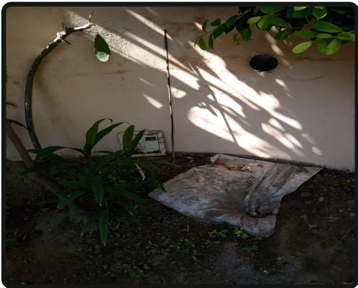
Roof top Rainwater Supply to Park
